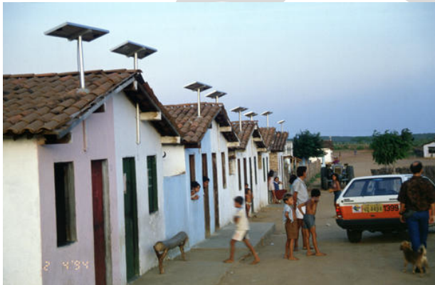
Brazilian homes use 50 Watt photovoltaic systems for lighting.
